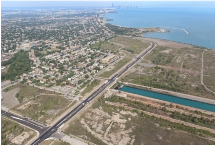
Stretching from 79th to 92nd streets, the two-mile extension of South Shore Drive cuts through the heart of the South Works site.
